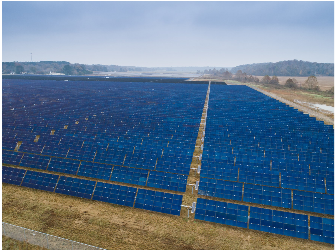
Silicon Ranch Solar Farm, Selmer, Tennessee
